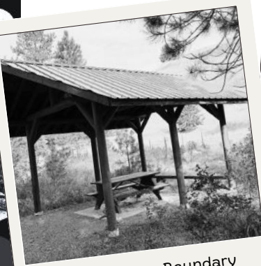
Metal roofing on Boundary Falls shelter
